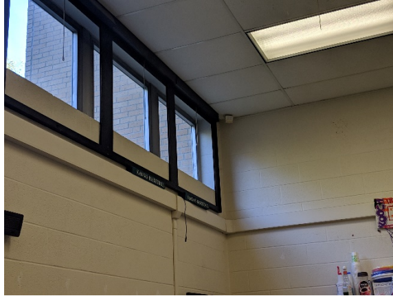
Figure 2.5 Corner of room scanned for initial 3-D lidar testing
